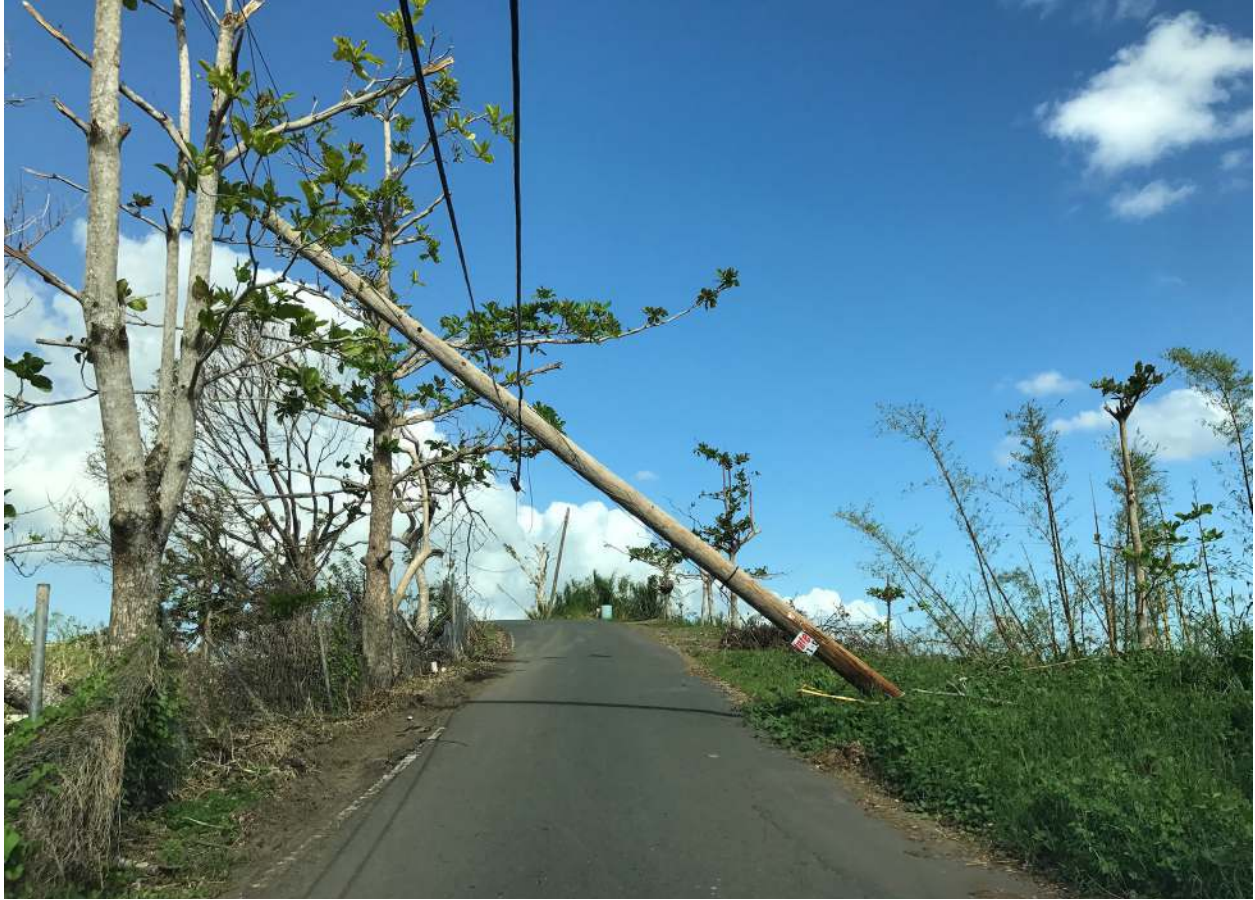
A utility pole resting on wires above a mountain road in Corozal, PR
