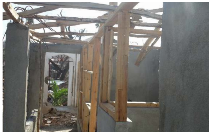
Figure 6 - Severely damaged studio
