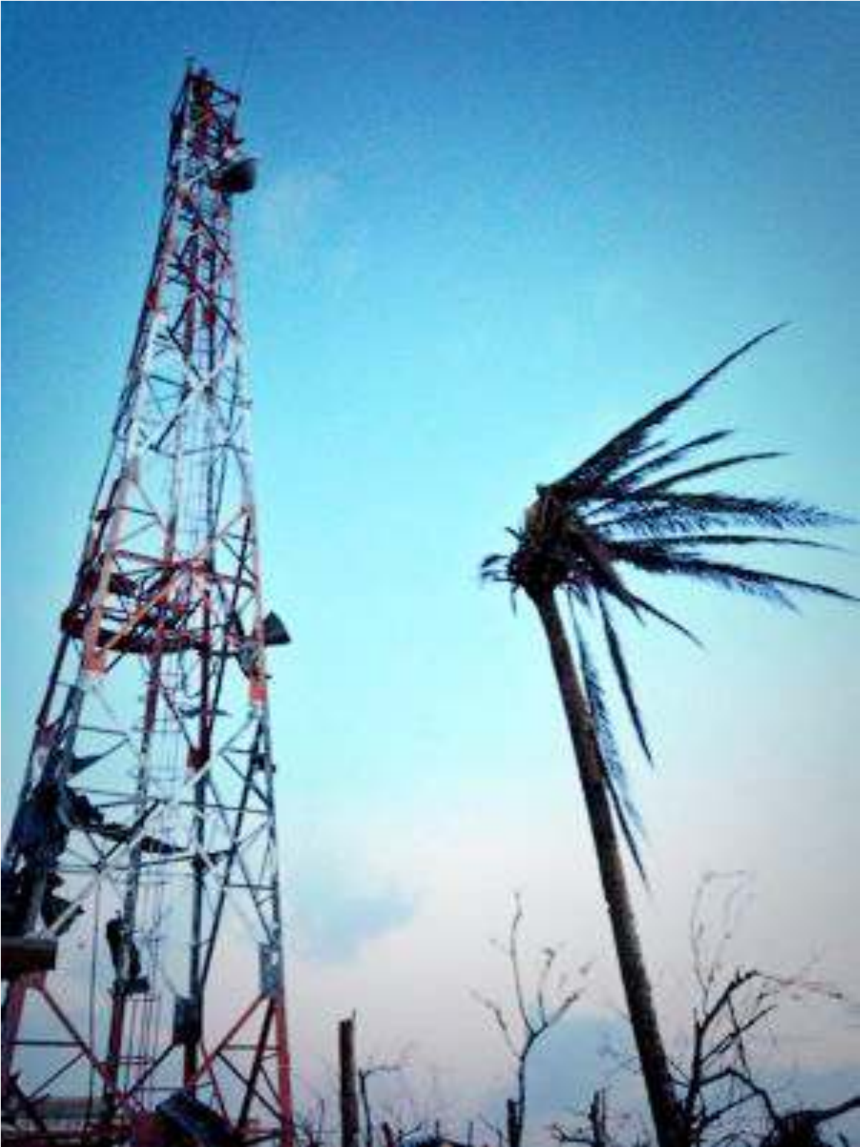
Figure 1: Telecom mast in Guiuan, Eastern Samar, later to be used to put up Radyo Bakdaw's antenna.
