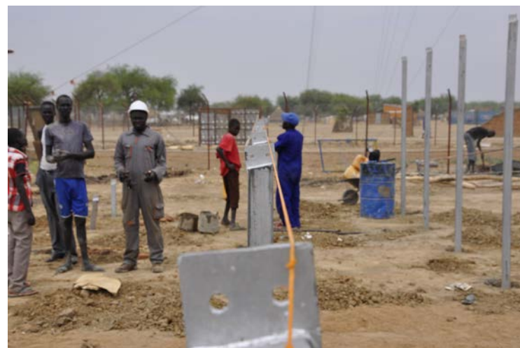
Figure 12 – Installing the mounting stands
