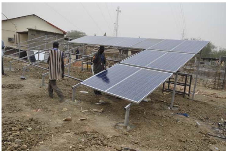
Figure 13 – Mounting the panels
